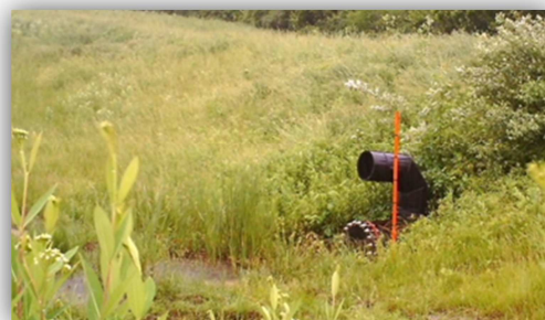
Figure 5-10: Detention basin retrofit technology cost-effectively optimizes excess capacity for downstream channel stability
